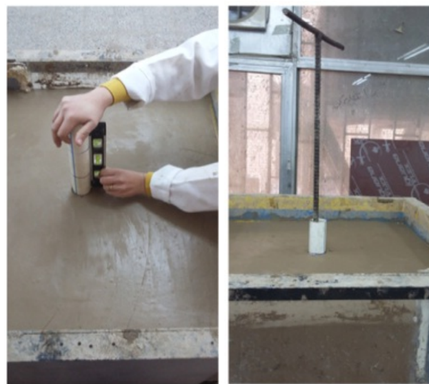
Fig. 4: The process of stone column installation.
