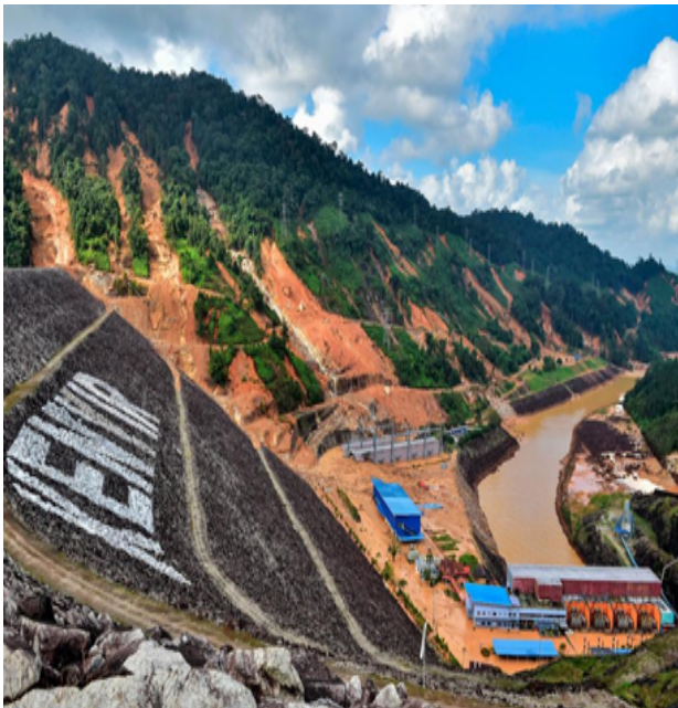
Fig. 1: Landslide that disrupted the accessibility to Kenyir Dam, Malaysia.
