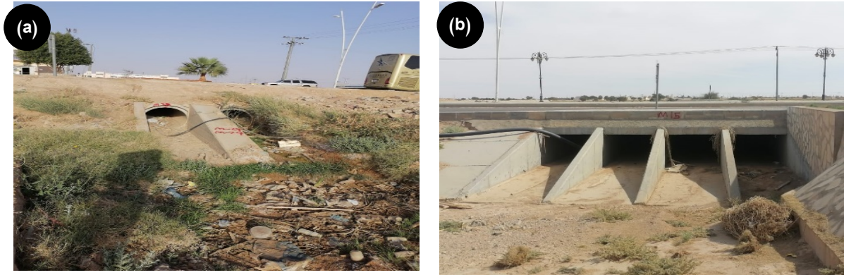
Fig. 26: sample of the existing culverts in the city of Al Bidi, where (a) a model for tube culverts, (b) a model for box culverts
