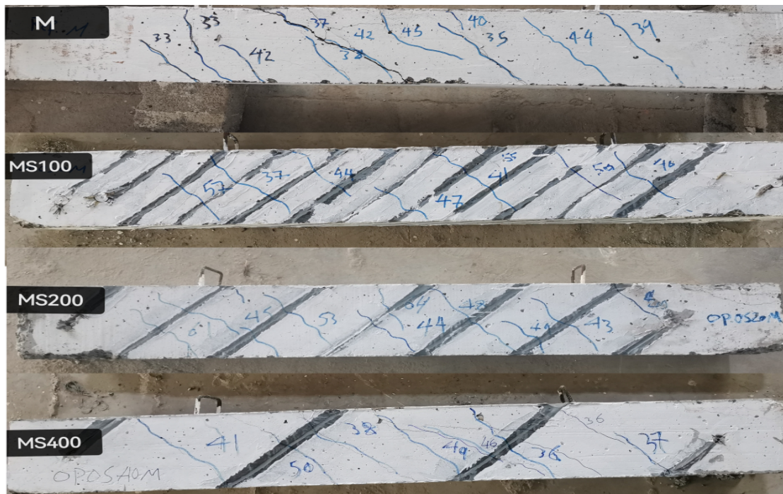
Fig. 14: Failure Mode for Beams under monotonic load
