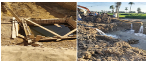
Figure 6. Increasing the level of water in the well.
