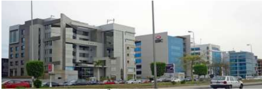
Fig.4: The southern 90 th street along with the office buildings.
