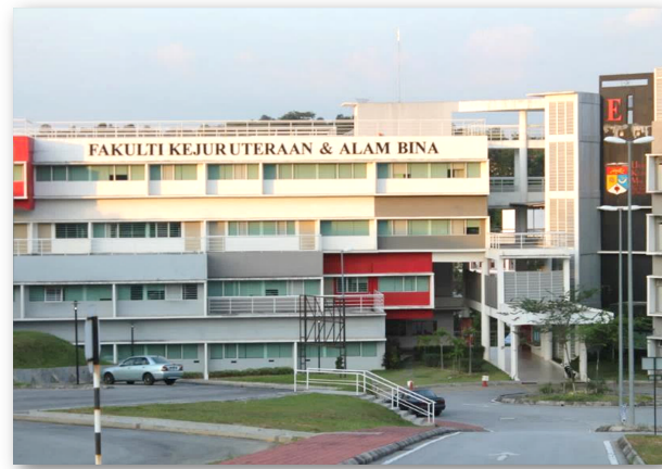
Fig. 2: High Voltage Power Laboratory in Universiti Kebangsaan Malaysia (UKM) Bangi, Selangor.
