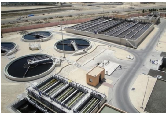
Fig. 1: Tubli Waste Water Treatment Plant [8].
